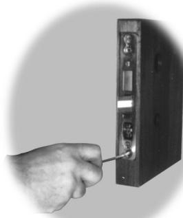
Insert lockbody (and hookbolts for Triad) into door prep. Check that lock fits easily in door with screw holes aligned. Secure lock to the door using lockbody screws. **Do not tighten fully at this time.**
