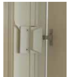
Sash Locks and Tie Bar Locking System
