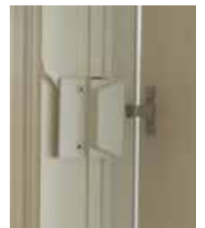
Sash Locks and Tie Bar Locking System
